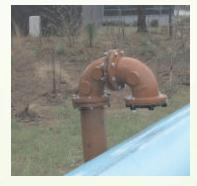
(a) Gas Production Plant (b) Water Pipe SOME APPLICATIONS OF FLANGE JOINT Fig. 5.12
